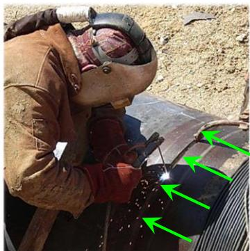
Magnetic and/or electric arc blowing
